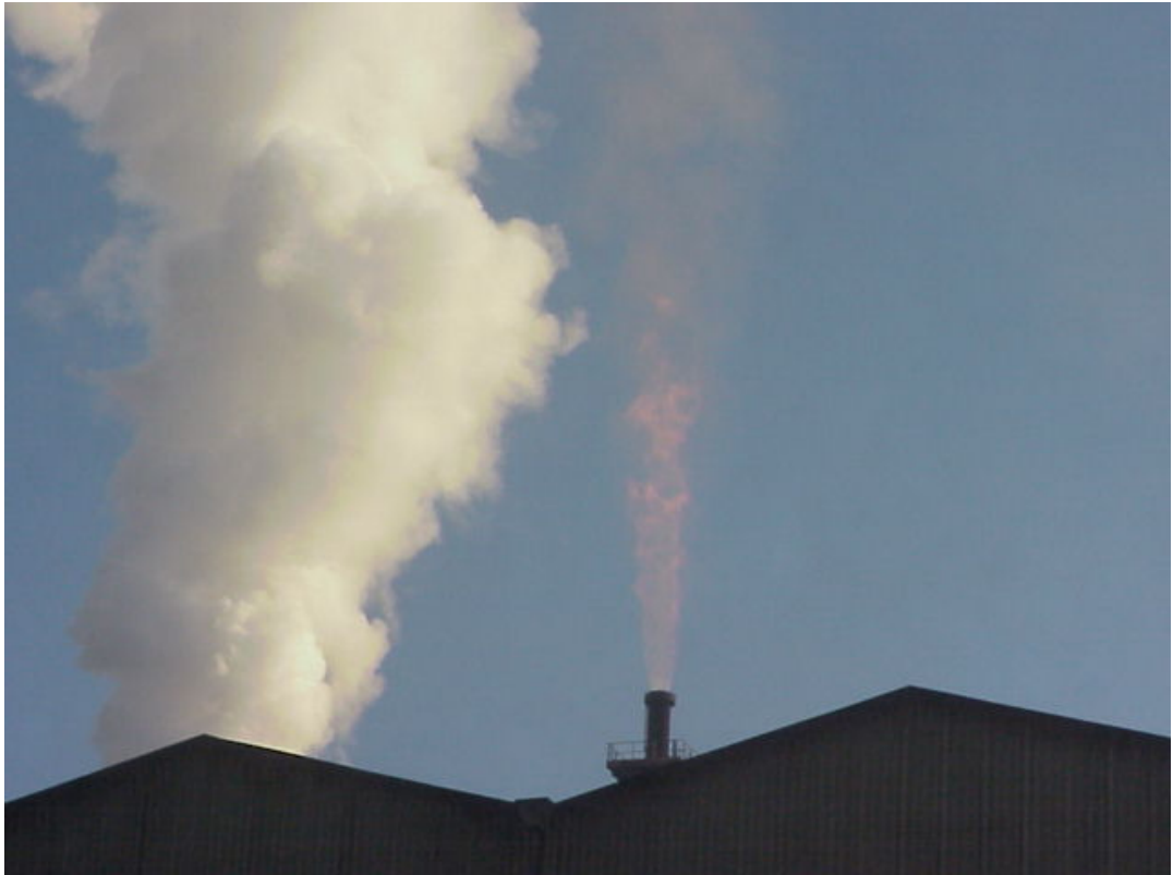
Photograph 1. KOBM Flare Stack
